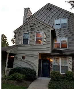
Private entrance on left leading upstairs.
